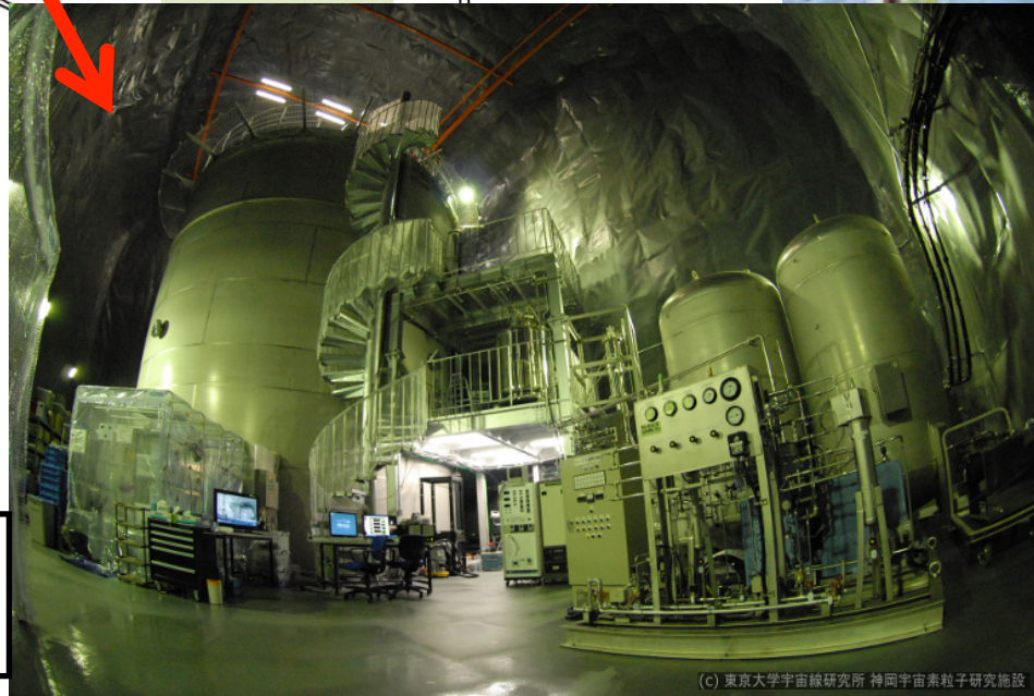
Kamioka mine Lab-C
